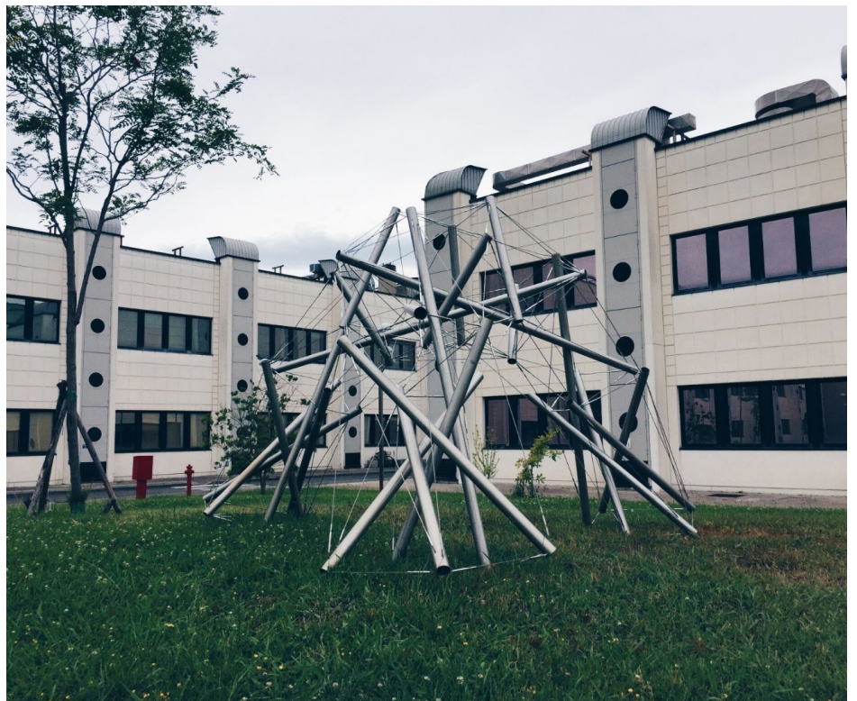
Fig 7. A full-scale manufactured tensegrity structure designed with the computational method developed at ISTI.
